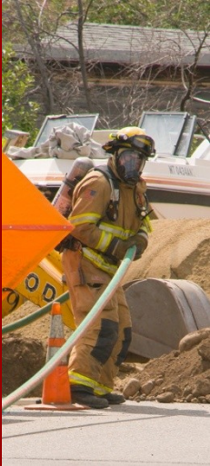
Firefighter Will Bernard pulls fire hose while operating on the scene of a natural gas leak.
